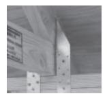
**Improvement 5** - Reinforcing roof-to-wall connections.
