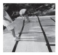
**Improvement 2** - Creating a secondary water barrier to prevent water intrusion. For example, using strips of "peel and stick-on" material that cover the joints between the plywood sheets on your roof to reduce leakage until repairs can be made if a hurricane blows off your roof shingles. There are two alternatives under Improvement 2:
