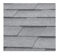
**Improvement 3** - *Improving the survivability of your roof covering.* For example, upgrading to stronger hurricane-resistant roof shingles, attached with properly sized and properly applied roofing nails, to reduce the susceptibility of your roof shingles blowing off in a hurricane.
